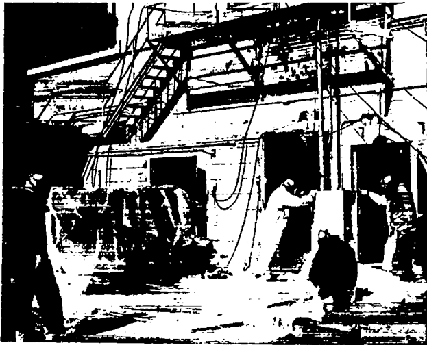
Fig. 10. Precipitron frame being rolled onto plastic sheeting.
