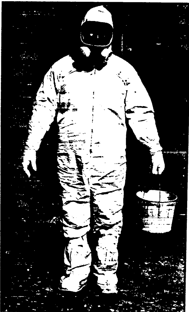
Fig. 34. Worker suited for demolition work.
